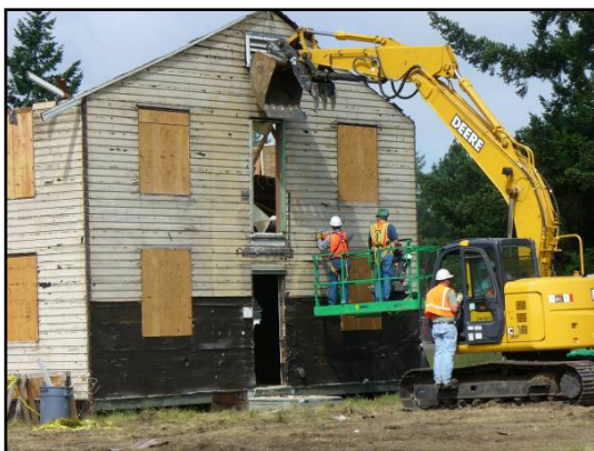
Left: Contractors prepare building for panelization, bringing the building down in partitions helped maximize recovery.
