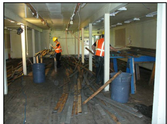
Left: Contractors prepare building for panelization, bringing the building down in partitions helped maximize recovery.
